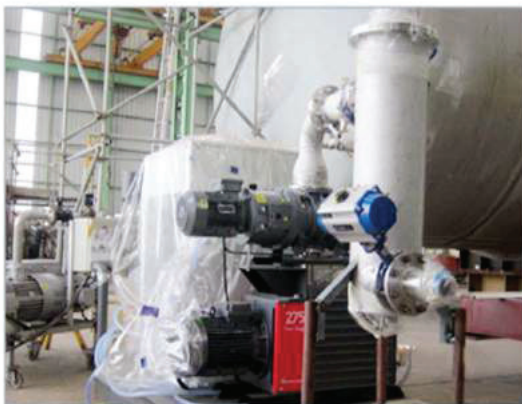
Vacuum pump w/ Booster E2M275 EH1200
