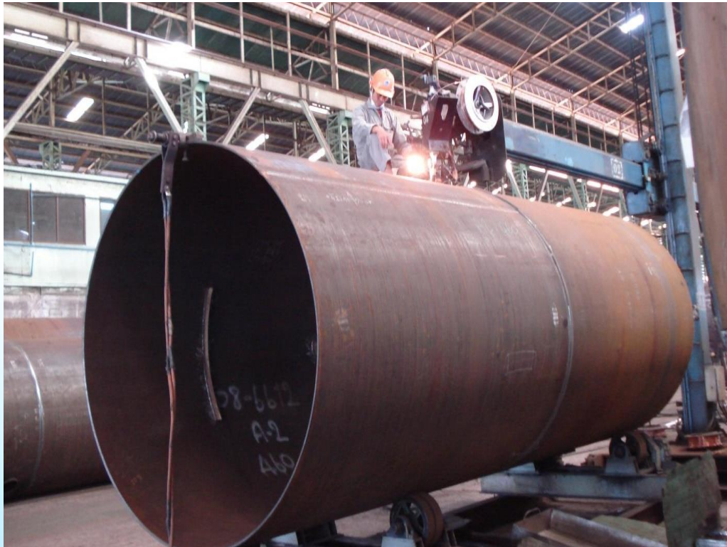
Semi-Automatic Longitudinal Welding with Manipulator
